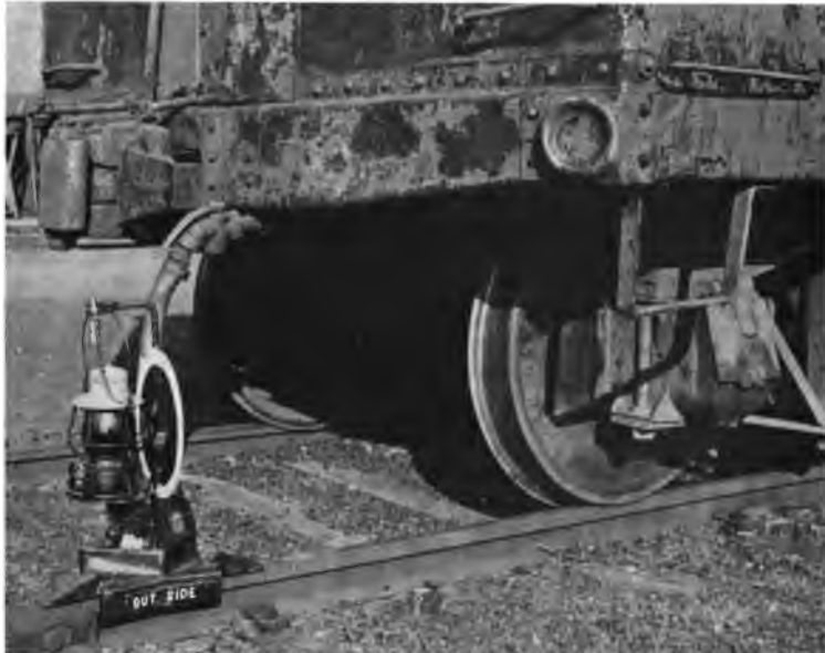
Fig. 3. Double Derailing Track Target. (National Tube Company.)*
